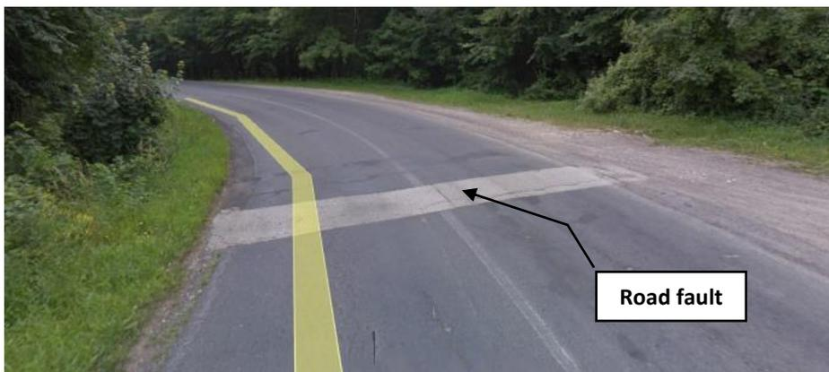
**Fig. 2.** Road fault causing a loss of stability
